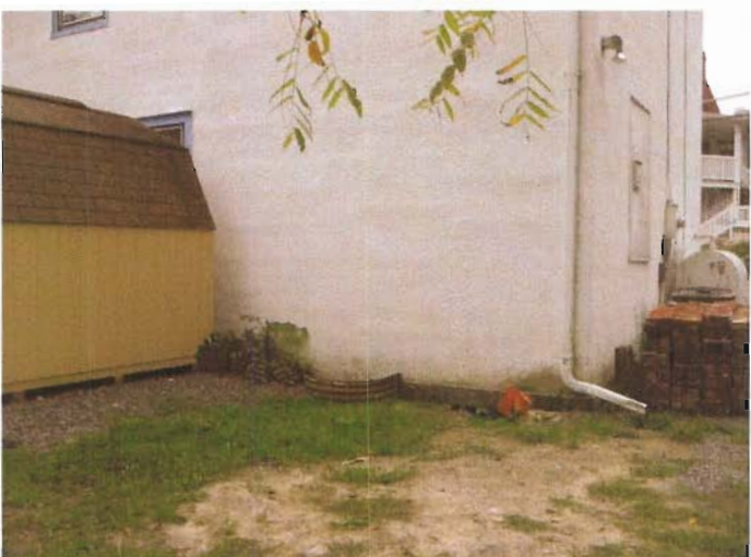
Side of Building
