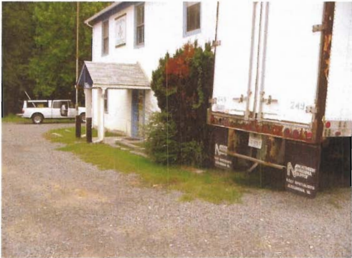
Front of Building
